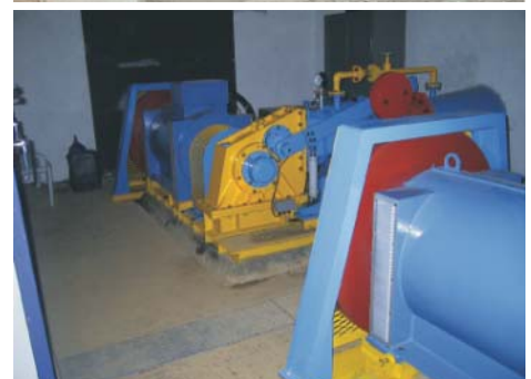
The electro-mechanical equipment features 2 x 125kW units. Turbines and all associated mechanical equipment was manufactured locally. The digital control system (DTC) was manufactured jointly by ENTEC AG and PT Heksa Prakarsa Teknik.
